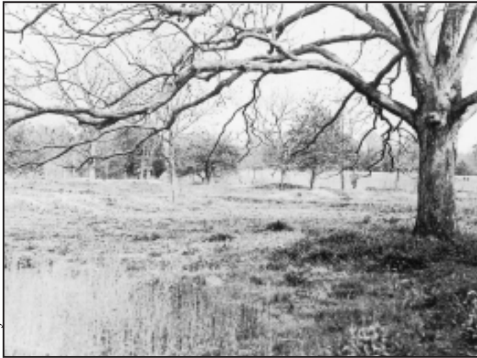
Pre-restoration photograph of east garden area.
