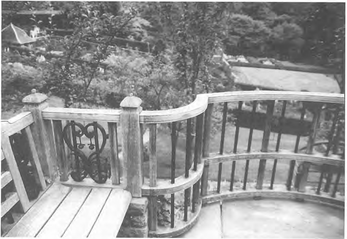
20. This detail of a bench that was constructed as an essential part of a railing at Dumbarton Oaks, Washington, D.C., illustrates Beatrix Farrand's remarkable facility with construction detailing and materials. S. Hollingsworth photograph.
